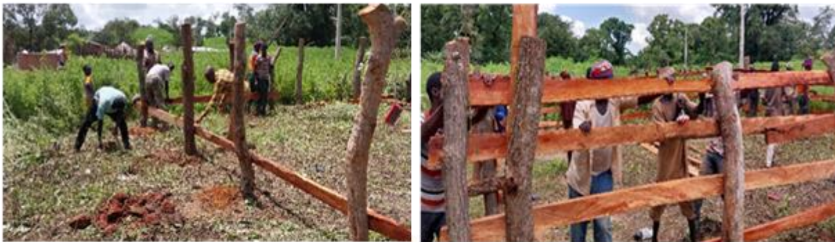
Community workers constructing the cattle night park in Sanzanou
