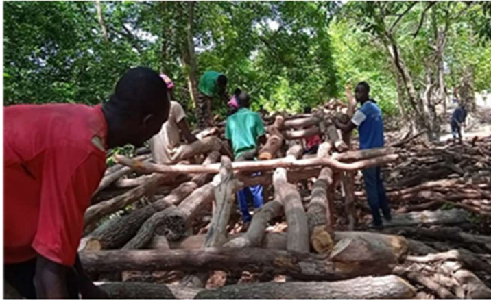
Community members choosing support beams
