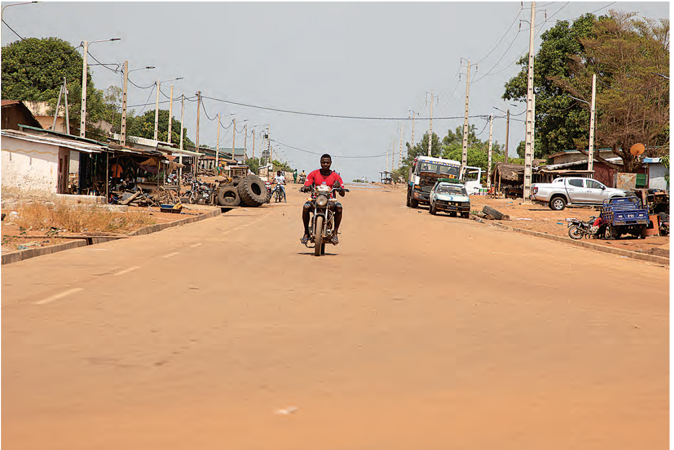
Crossroads former regional council of Minignan leading to the different border tracks
